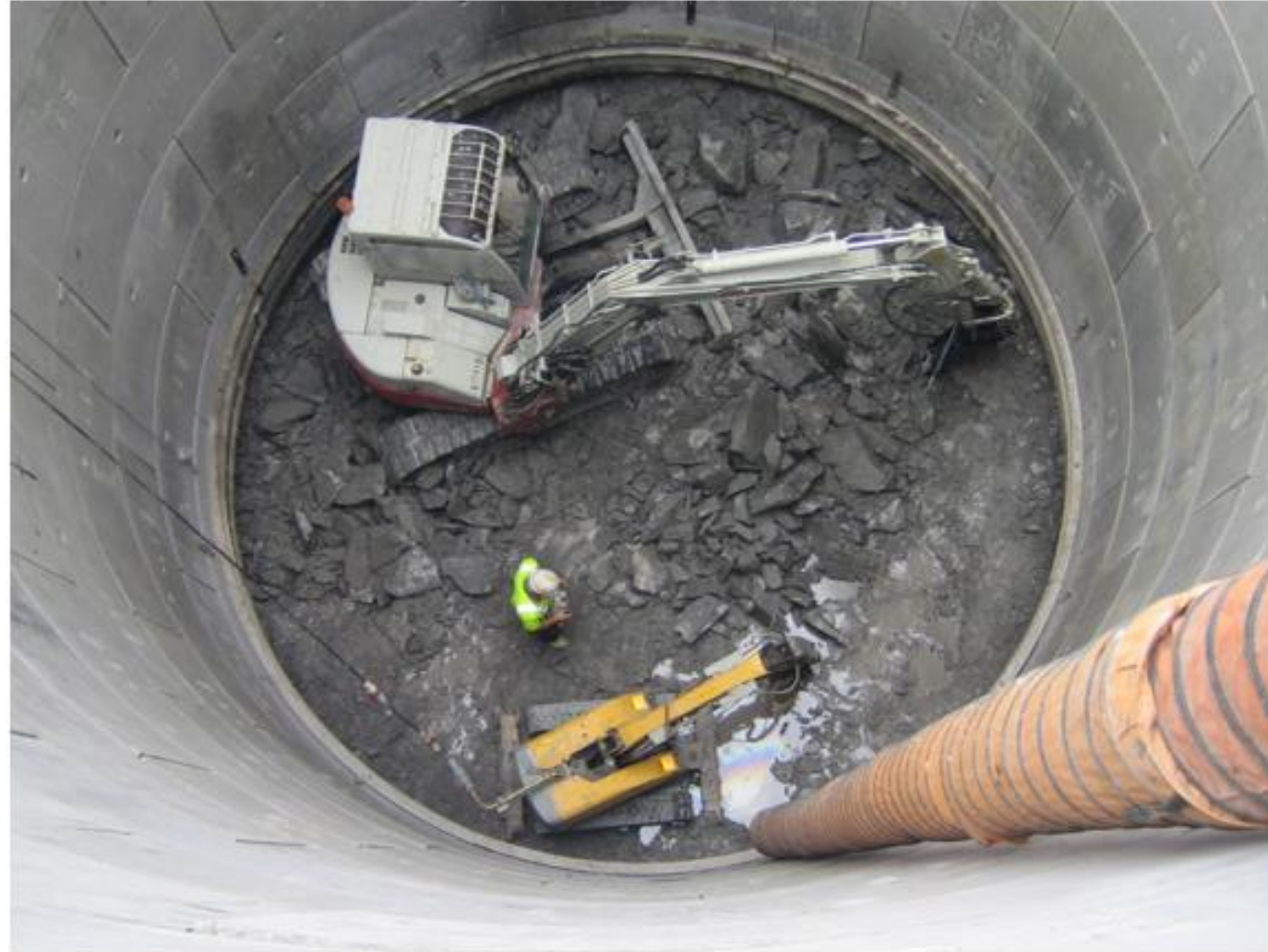
Brokk 160 (1.6 Ton) and TB180 (8 Ton) Size Comparison in Shaft Sinking
